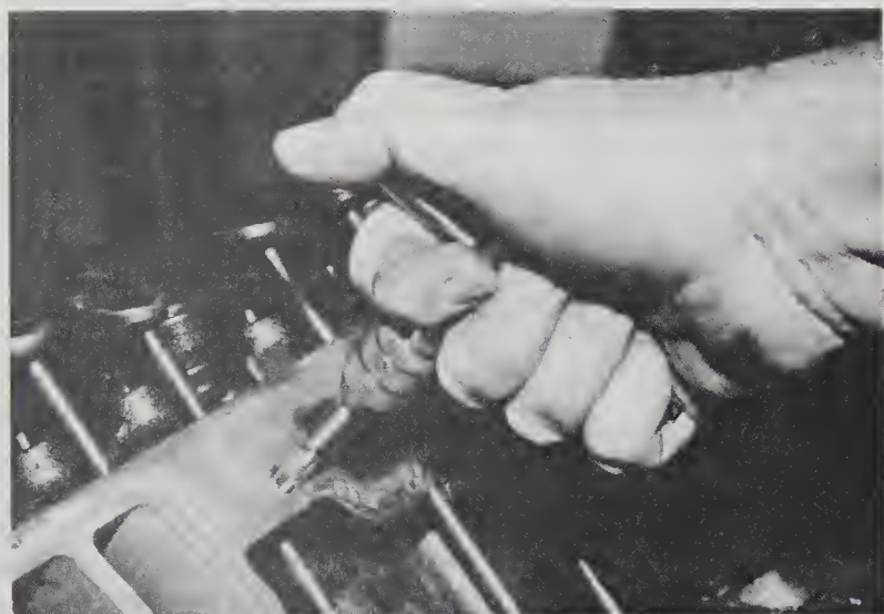
8.5a Run a tap into all threaded holes to remove old sealer, rust and scale
