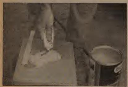
5 Following label instructions, mix up a batch of plastic filler and hardener. The ratio of filler to hardener is critical, and, if you mix it incorrectly, it will either not cure properly or cure too quickly (you won't have time to file and sand it into shape)
