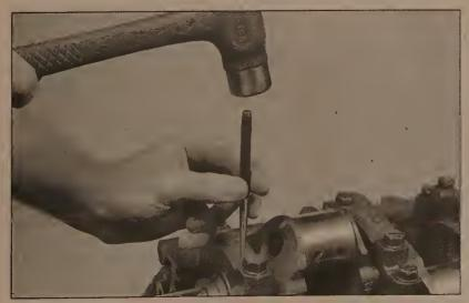
13.4a Use a center punch or number stamping dies to mark the main bearing caps to ensure that they're reinstalled in their original locations on the block (make the punch marks near one of the bolt heads)
