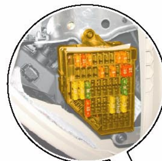
Fuse box, in right-hand side of dash panel
