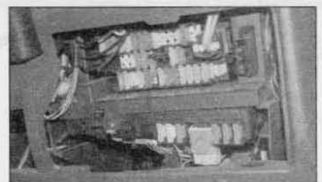
E Check that all fuses are still in good condition and none have blown.
