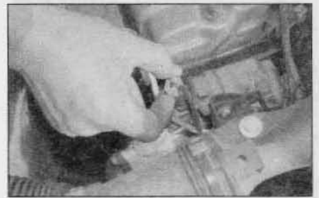
C Also check the security of the wiring connectors at the various engine management sensors such as the coolant temperature sensor.
