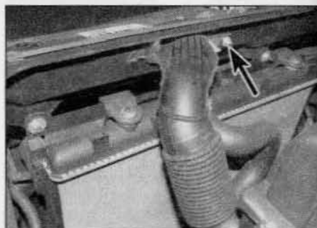
2.8 Undo the nut (arrowed) securing the air intake duct to the front body panel – later models
