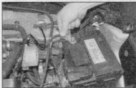
A Check the security and condition of the battery connections.
