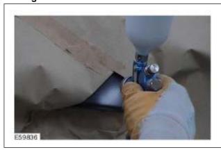
The filler layer is applied in stages. First of all, filler is only applied to the location which has been sanded away. After a wait time for flashing off, the second coat is applied so that it spreads over onto the existing paintwork.
