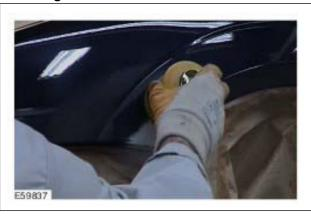
The repair location is now rubbed down with P400 - P500 and the bordering surface with P2000 - P4000. Remove sanding residues and clean the repair area with silicone remover.
