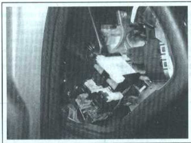
3.1f . . . there's a fuse panel under the cover
