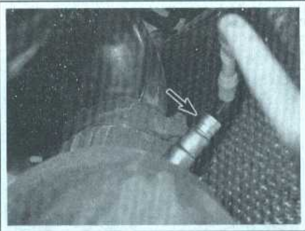
13.9a The right upstream oxygen sensor (shown) and the left upstream oxygen sensor (not shown) are located on the exhaust pipe right below the exhaust manifold flange and right above the upper end of the catalytic converter (V6 models)
