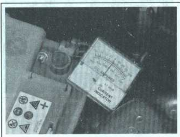
13.3 Use an inductive ammeter to measure starter current draw
