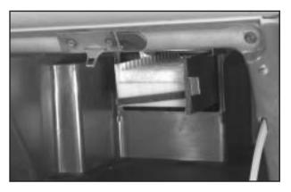
2. Then push the tab, located on the left of the inner access panel, to the right.
