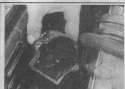
Fig. 24 Once removed, check the cap carefully for damage and wear. If its condition appears marginal, it is always a safe decision to simply replace it
