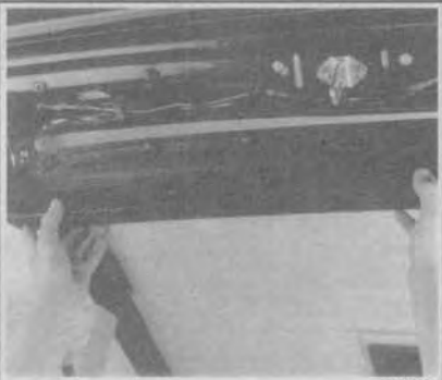
86836723 Fig. 57 Removing the panel to expose wiring and motor
