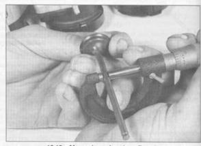
12.18a Measuring valve stem diameter
