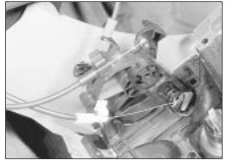
9.5 Removing the heater control panel
