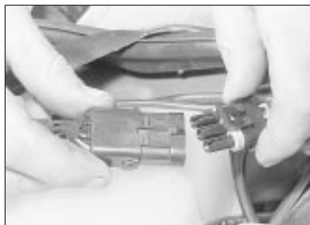
12.94 Disconnecting the oxygen sensor multi-plug
