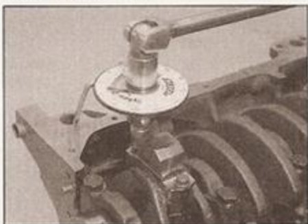
13.22 ... and Stage 2 torque settings
