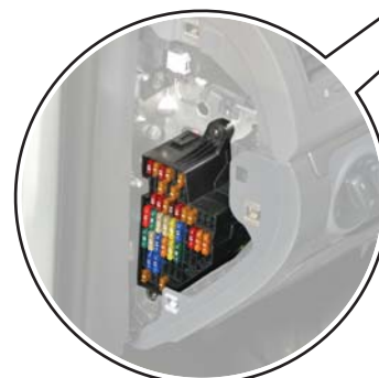
Fuse box behind the instrument cluster
