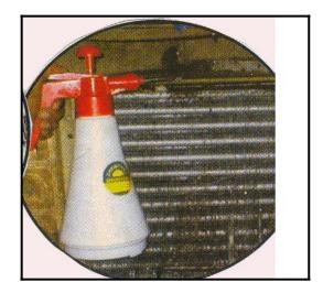
4. After Spraying, the Liquid becomes Foam & enters in the Evaporator coil.
