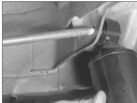
16.2a Removing a shock absorber upper mounting ...
