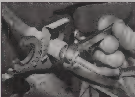
12.4b Slacken the brake pipe union ...
