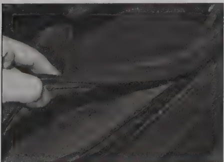
24.14 Pull back the door seal from along the sill trim panel
