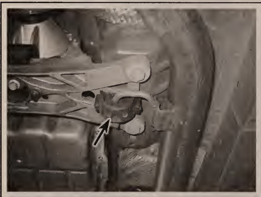
18.2 Inspect the hangers for signs of deterioration
