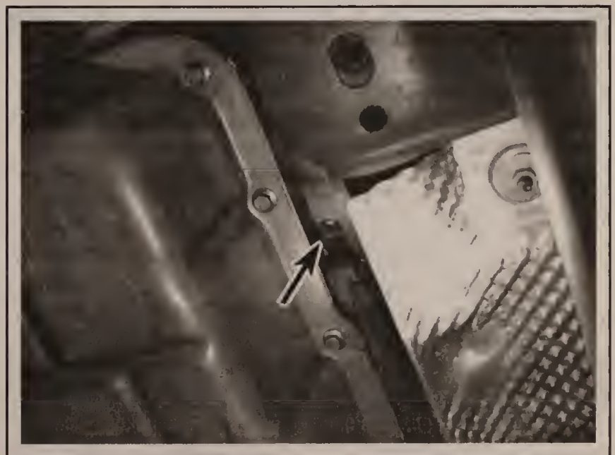
13.1 Look for the evaporator drain hose under the vehicle above the transmission on the right side
