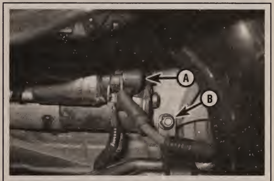
4.4b The third battery cable (A) is connected to the B+ terminal on the starter motor solenoid. The engine ground cable bolt (B) is also located near the starter motor
