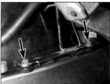
13.3 Unscrew the bolts (arrowed) and detach the hose guide
