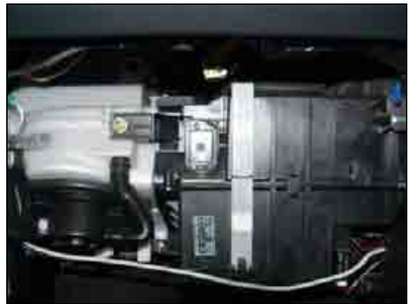
After the filters are installed
