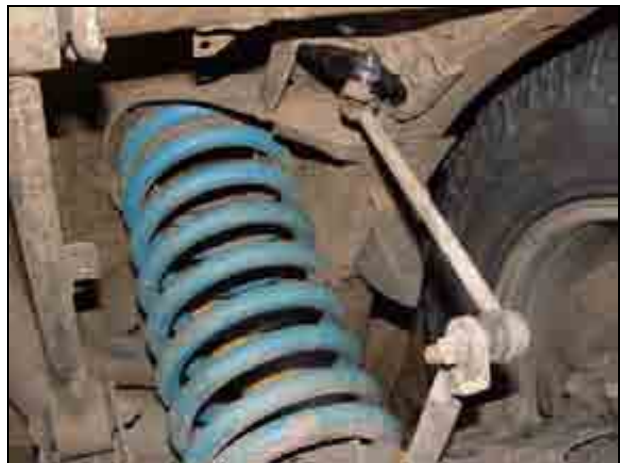
Left hand bracket installed
