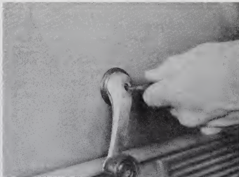
9.3 Use an Allen wrench to remove the window crank
