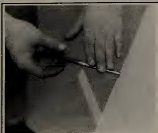
Fig. 139 Valve stems may be rolled on a flat surface to check for bends
